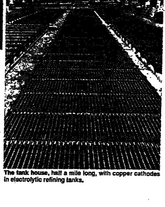
The tank house, half a mile long, with copper cathodes in electrolytic refining tanks.
